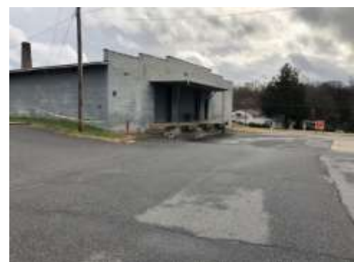
Existing building west loading dock elevation
