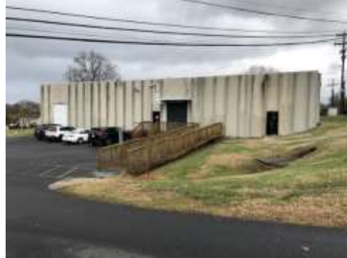
Existing building corner of Sloan & Depot Streets
