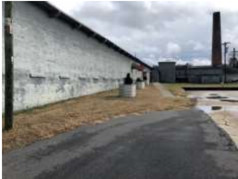
Existing building south elevation
