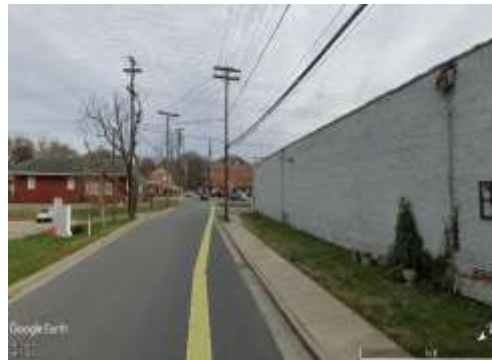
Existing building Depot Street view
